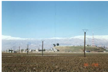
Overhead Lines in the Beqaa Valley
